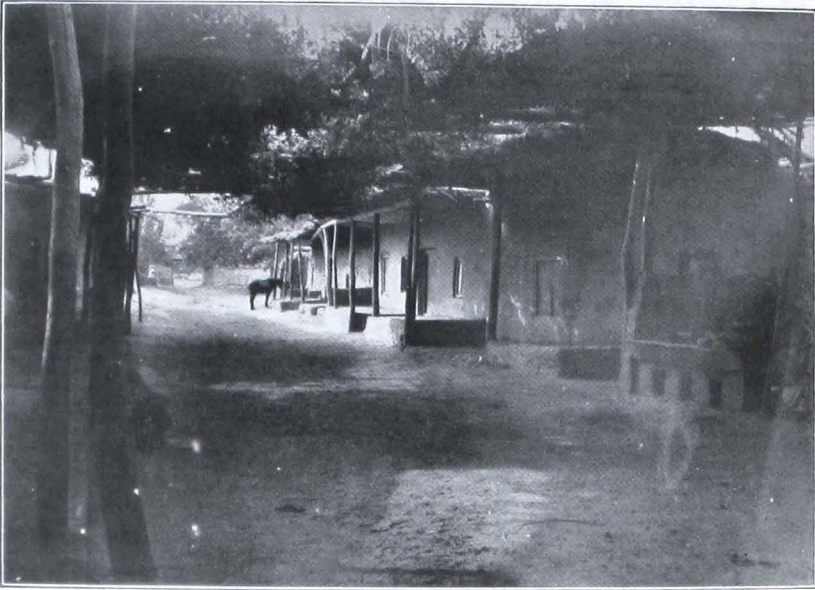
A Roofed bazar street, Bugur
